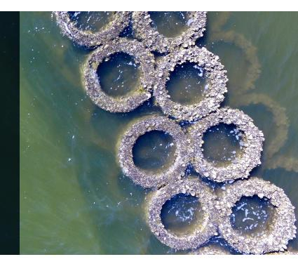
The patented Natrx Oysterbreak is a breakwater system designed to support coastal protection through a high-strength modular design and special material additives to support biological growth.
